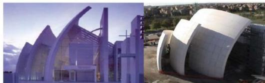
**Fig. 2:** A view of the church Dives in Misericorida made with cement with self-cleaning capability.
