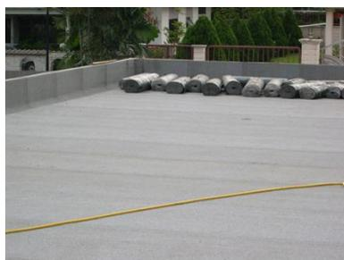
**Fig. 1:** The self-protected membrane waterproofing system.
