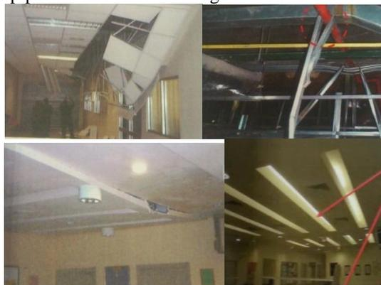
**Fig. 1:** Ceiling collapse at suspended ceiling and hair line cracks and sagging at plaster ceiling
