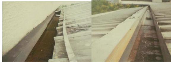
**Fig. 3:** Corrosion at the roof gutter
